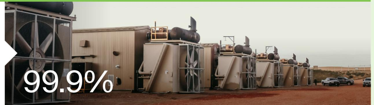
Crusoe's DFM™ technology converts the natural gas captured at oil wells and converts it into electricity by leveraging a stoichiometric combustion process, which allows reaching a 99.9% methane destruction efficiency.
